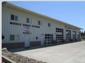
Middle Grove, Station #2
